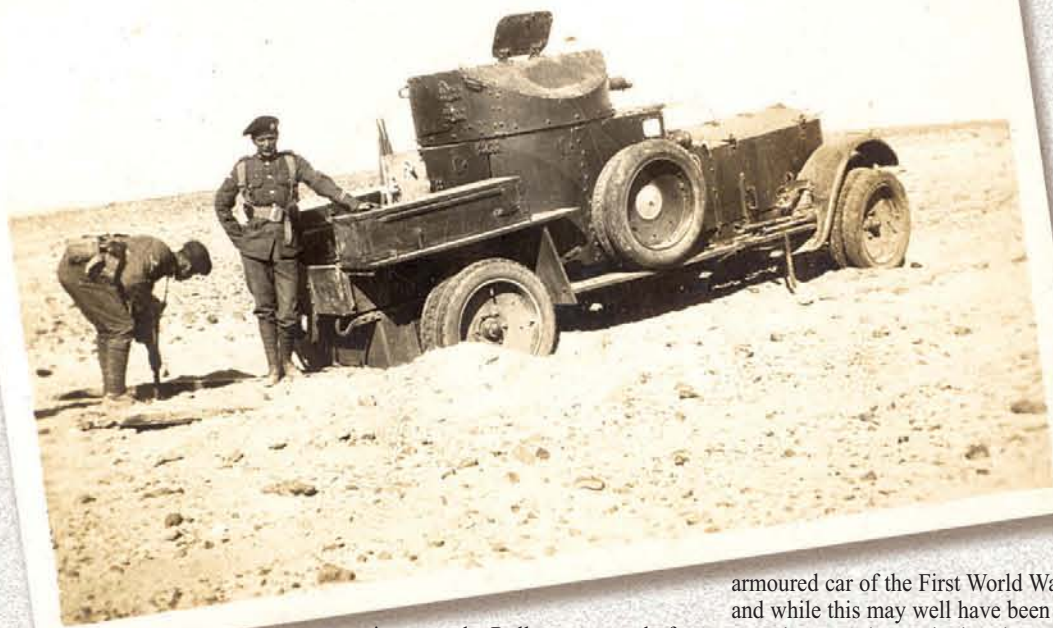
Above: the crew have fitted double wheels on the front axle to help get through the sand - sadly without success! (Photo - James Payne)
